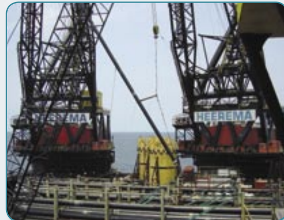
Tendon sections are upended and joined aboard the Thialf .
