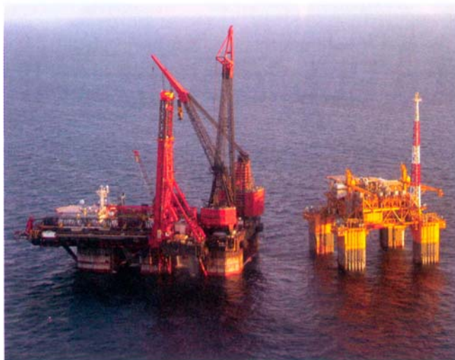
Figure 2. Balder works on Independence Hub.
