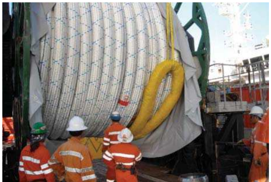
Preparing to spool polyester rope onto the MLDW. All photos courtesy Shell.
