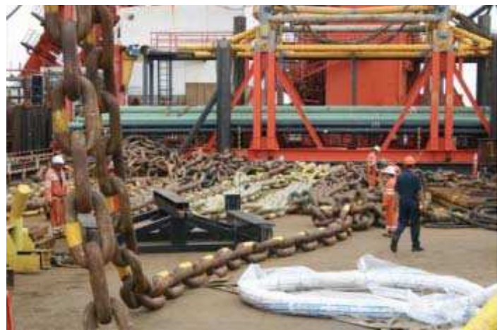
(Above) Connecting sections together with H-links. (Below) Handling chain.
