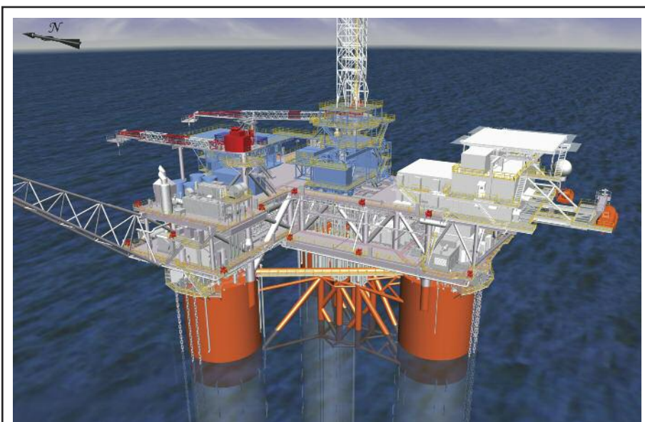
ATP Oil & Gas Corp.’s Telemark Hub is deploying the ATP Titan—the Gulf’s first minimum deepwater operating concept (MinDOC)—to initially produce two dry tree wells at the Mirage Field in 3,927 feet of water at Mississippi Canyon 941, one or two dry tree wells at Morgus in 3,960 feet of water at Mississippi Canyon 942, and a subsea well tied back 11-12 miles from the Telemark Field in 4,385 feet of water at Atwater Valley 63. In the second phase of development, the ATP Titan will move from Mississippi Canyon 941 to Atwater Valley 63 to drill additional wells at Telemark.
