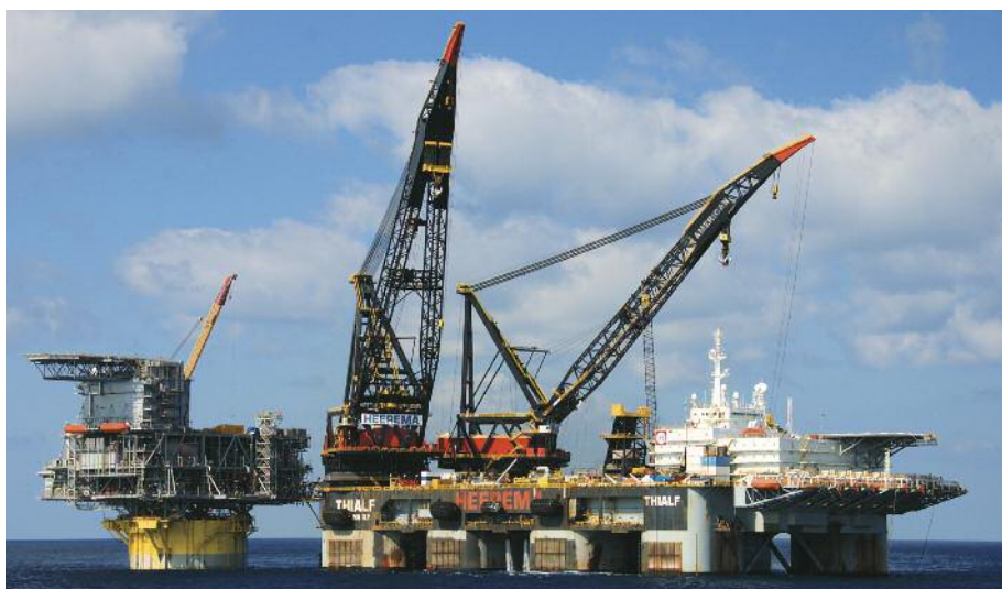
Shell's Perdido Hub Development in the Perdido Foldbelt is establishing first production from the Lower Tertiary play using a direct vertical access spar stationed in nearly 8,000 feet of water to produce wells in up to 9,627 feet of water. The spar was installed late last summer and the topsides were mated to the spar in mid-March using a single lift of Heerema Marine Contractors' Thialf heavy-lift vessel. Shown here, from top to bottom, is the Thialf arriving on location, installation of the living quarters/helipad, and the spar with all topsides facilities in place. Initial production is planned for early 2010. Photos courtesy of Shell and Jan Berghuis Terschelling, captain of Heerema's Retriever .
